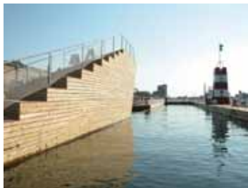
stage e passerelle temporanei
